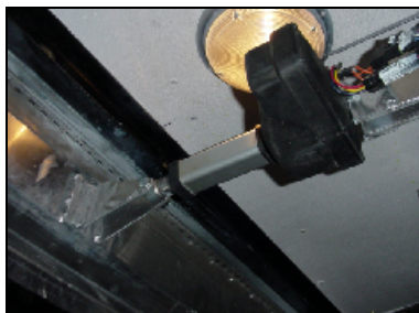
Damper with linear actuator – interior view
