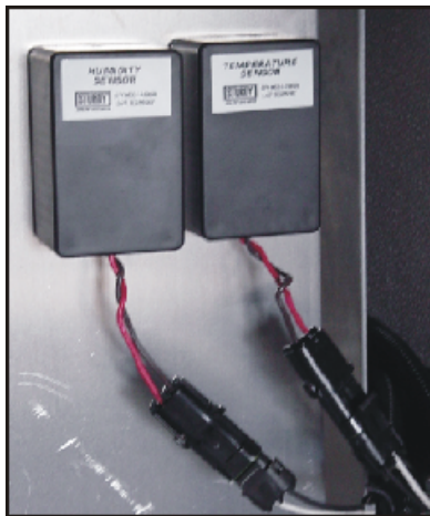
LEFT: Interior mounted Temperature & Humidity Sensors
