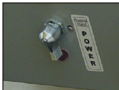
Electrical Control System Master Disconnect
